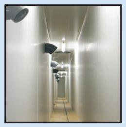
Plenums serve the double purpose of helping to maintain a consistent negative pressure pulling spent air from the hatcher and allowing a place for easy clean-up of accumulated airborne debris.
